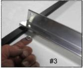
Then roll the rails over so the bolts slip into the holes on the panel frame. Place the flange nut on your finger with the flange UP and thread onto the bolt from underneath as shown in Photo #3. Finger tighten.
