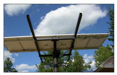
Center rails on longitudinals by equally measuring side to side to longitudinal ends. Then place the rest of the panels on the rails. NOTE: Leave the bolts on the PV panels screwed together but loose for now.
