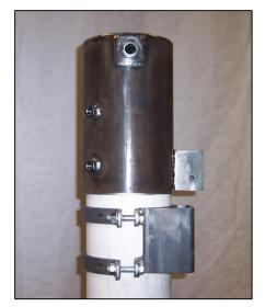
Place pivot cap on top of steel post. Orient pivot bore with bronze bushings east and west. The 4 set bolt nuts should face south. Secure the pivot cap with  $\frac{3}{4}$ " square head set bolts.
