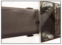
longitudinals (2 ½" sq. washer on top, 3" sq. washer on bottom) with 8" bolts. When both longitudinals are installed, tighten the
