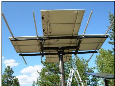
Repeat rail attachment procedure on left and right until all remaining panels are installed. When all panels and spaces are square and even to one another, tighten stainless steel panel bolts and all u-bolt nuts.
