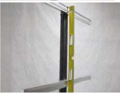
Hold a level on centerline as shown. Note bubble. Now move level to outer end of channel next to brackets. The bubble on the level must read the same; this will ensure that the panels are in plane. Now tighten the U-Bolts. If the channels are not in plane then you will have a twist to your panel(s).
