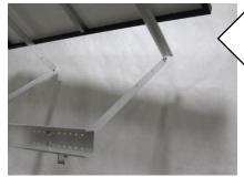
Attach braces to bottom of panel rails as shown at left.
