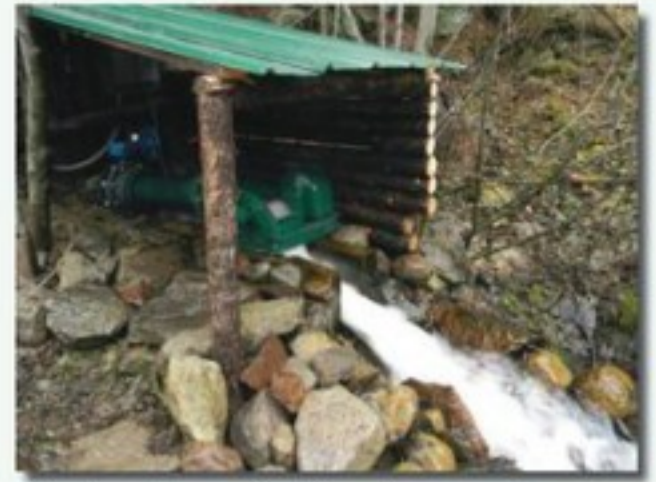
No dam is required, only an upstream diversion through a 6" pipe, which is coupled to the unit.
