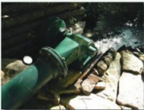
A low-RPM permanent magnet generator is direct-coupled to the turbine.
