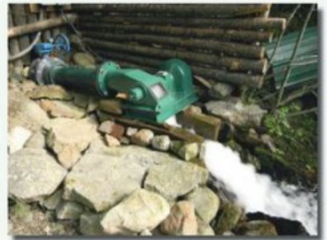
No dam is required, only an upstream diversion through a 6" pipe, which is coupled to the unit.
