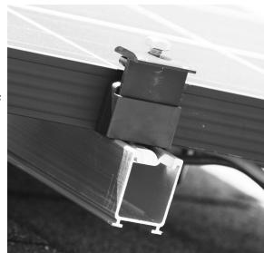
Place the first module onto the rails so that it is centered over the rails. Make sure the module is touching the inside edge of the clamps and tighten the clamps with a 1/2" socket.
