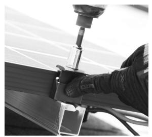
Install 50-50 Clamps in each rail on the other side of the first module. The springs will hold the clamps in place prior to tightening. Place the second module on the rails, align it with the first module, and push in against the clamps. Tighten the clamps to fully secure the module.
