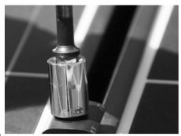
Insert channel end clamp in the rail. The module must be lifted slightly to slide the clamp under the frame.
